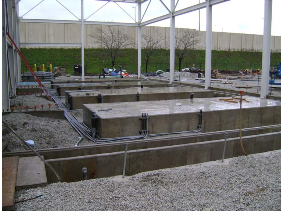
Engine-Generator Equipment Pads
