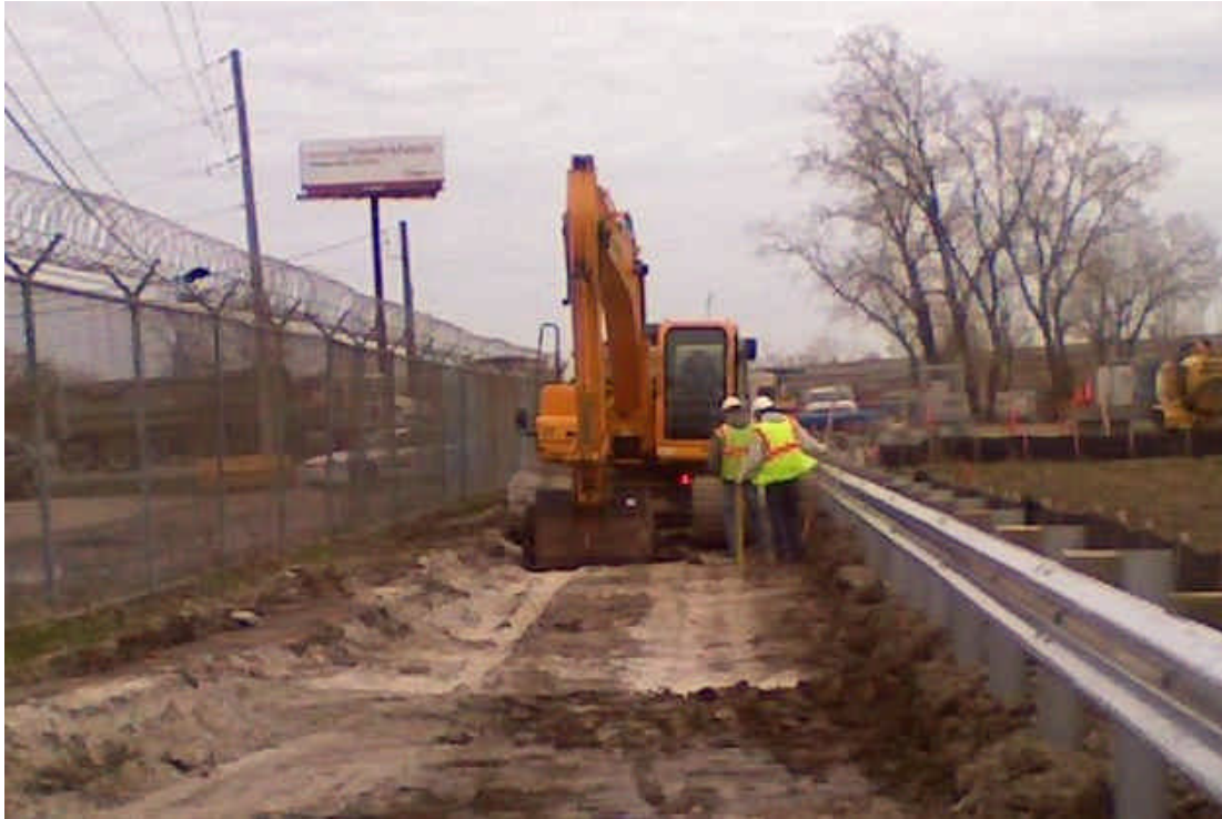
South Road aggregate placement
