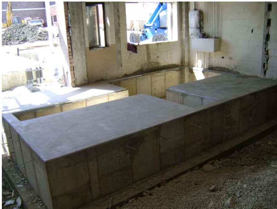
Day Tank Fuel Containment in Existing Service Building
