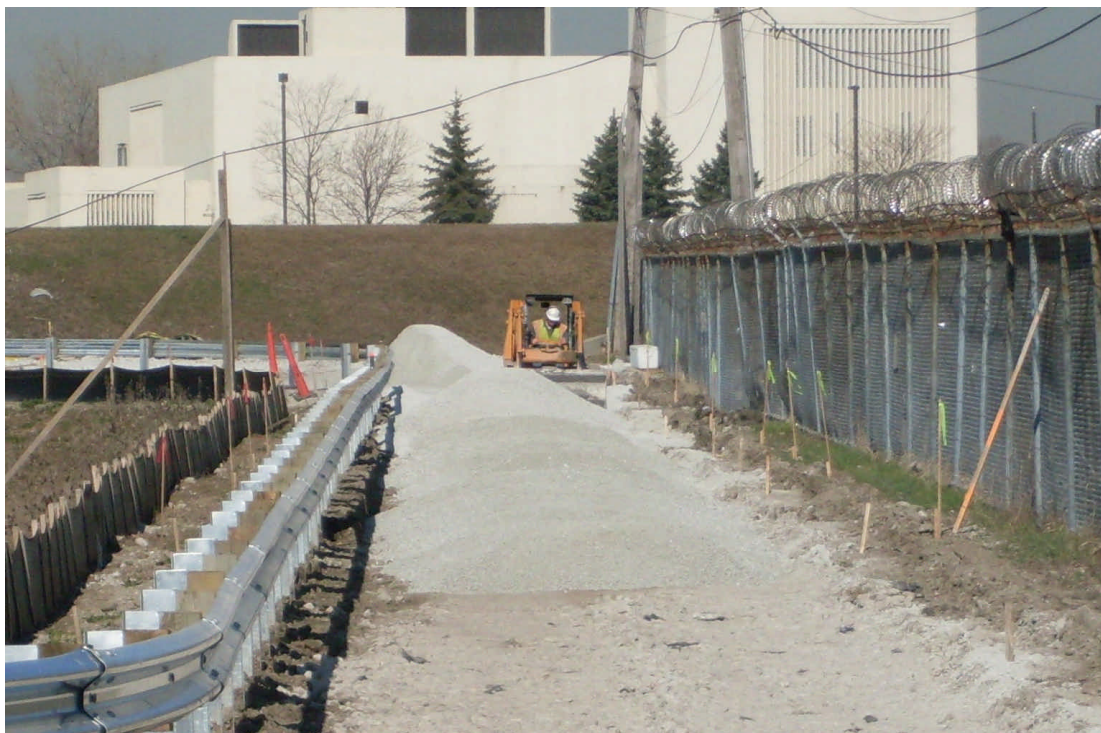
South Road aggregate placement
