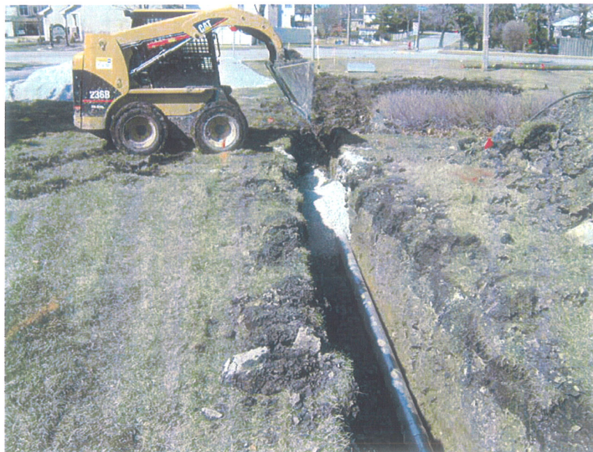
Installation of 5" Steel Conduit for Electrical Service to Plant
