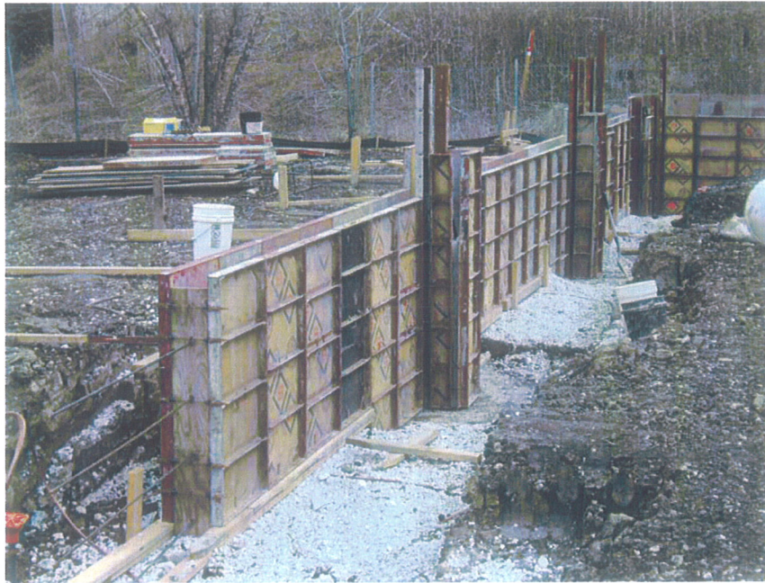
Office Building Foundation Construction
