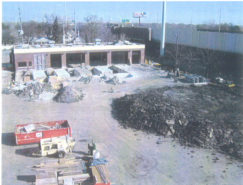
Overview of Generator Building Progress
