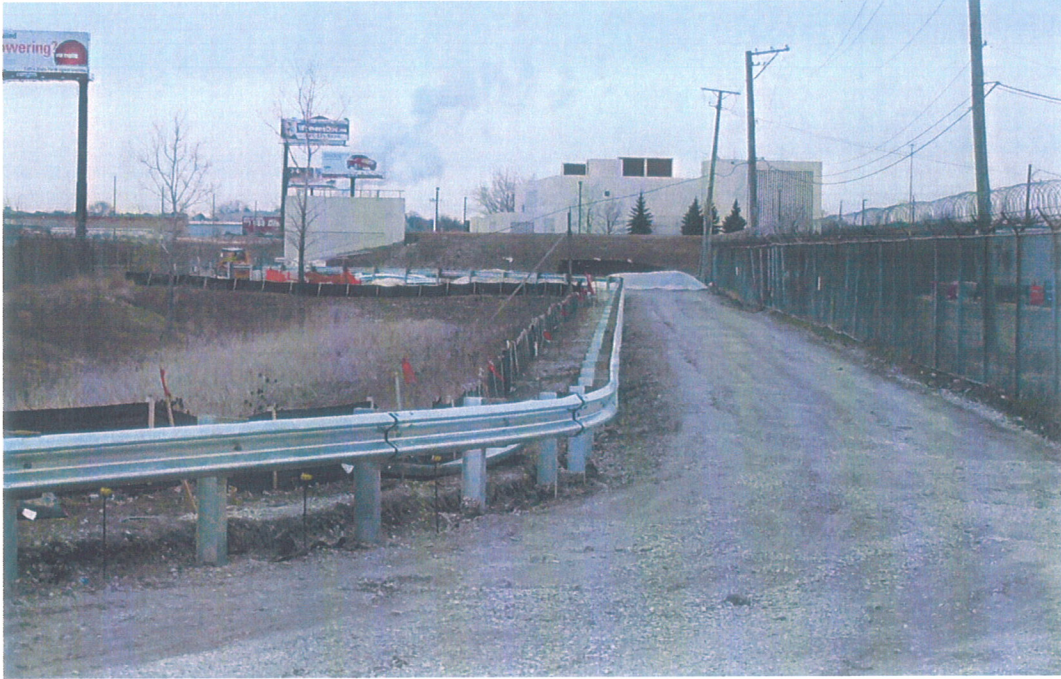
South Access Road guardrail installed
