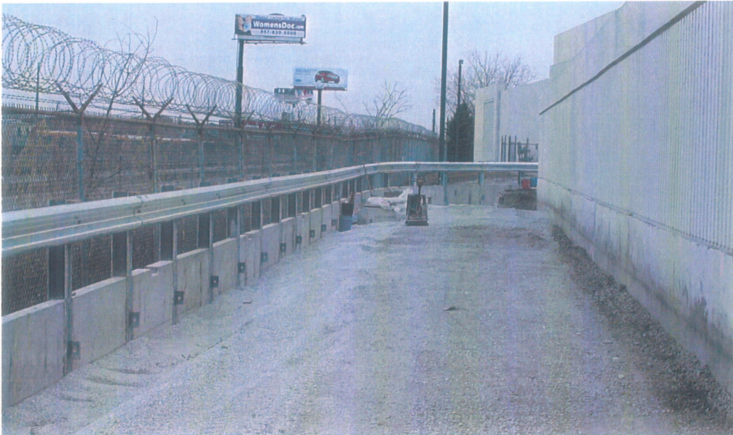
Soldier-pile wall with guardrail
