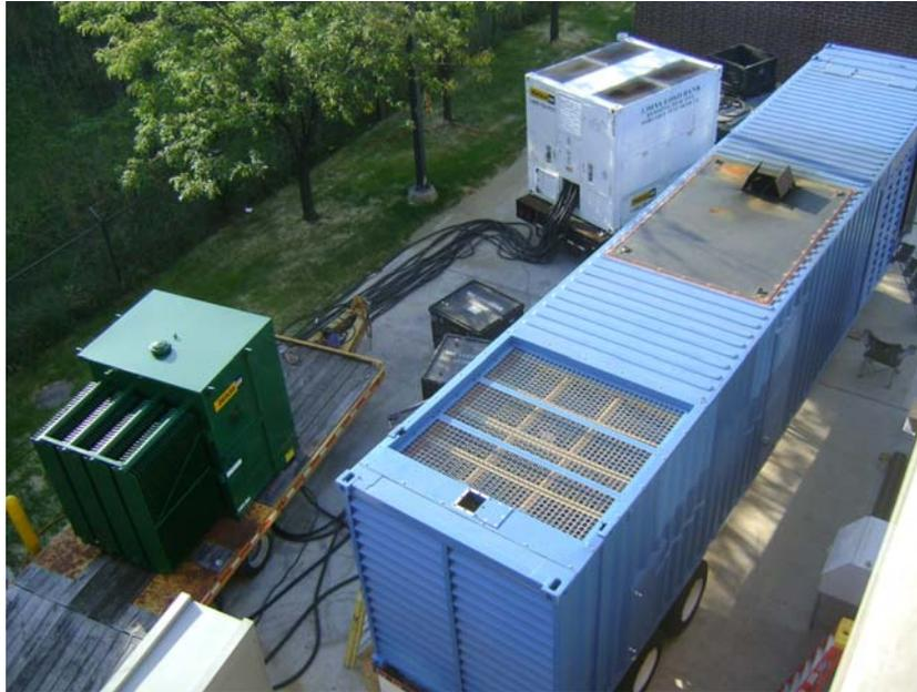
Portable Generator and Generator Testing Equipment
