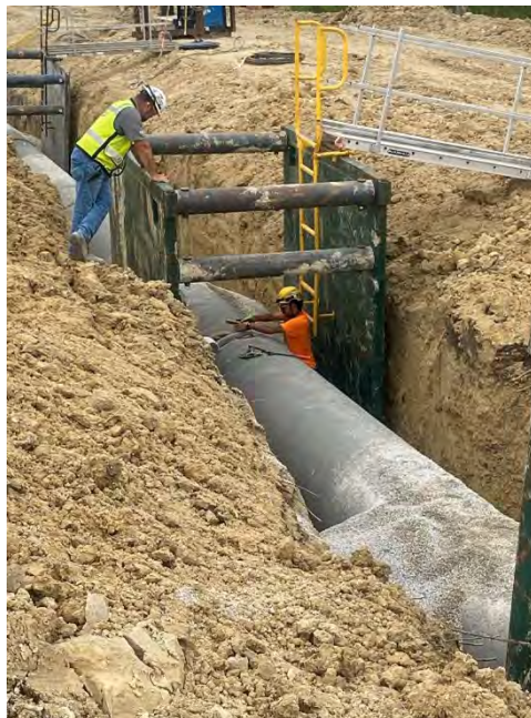
36" Bar Wrapped Pipe, External Joint Coating, Diaper Installation
