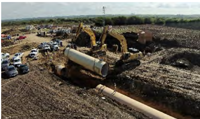
Section 12-13-MBR – Installation of 108-inch welded steel pipeline
