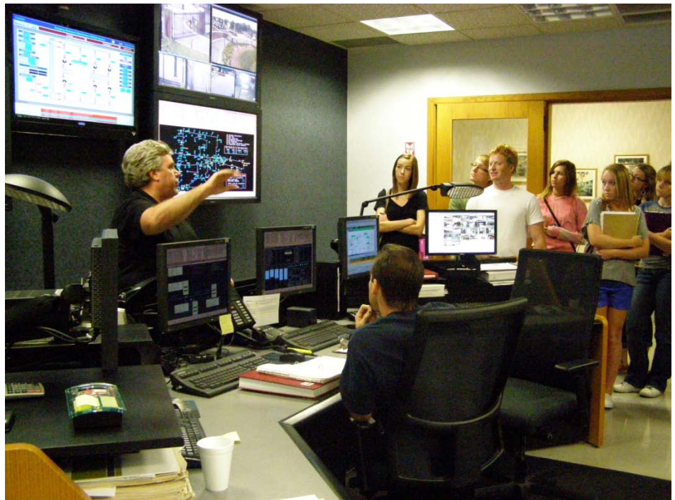
McGhee explaining how the control room works
